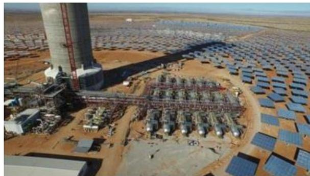
Figure 10: Steam accumulators in Khi Solar One.
