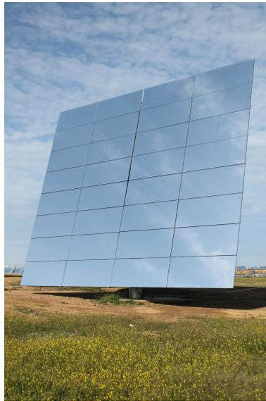
Figure 2: Abengoa heliostat with 8x4 facets.
